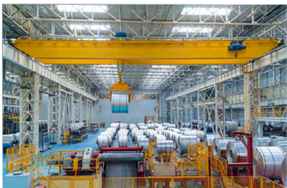
Skewing can occur in particular due to load swing, which subjects crane wheels and rails to increased strain and wear.
